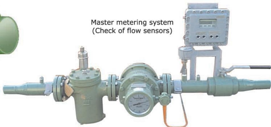
Master metering system (Check of flow sensors)
